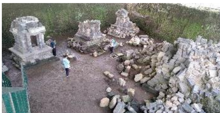
Figure 12. Losari Temple in the district. Salam is one of the temples that collapsed due to natural disasters and was buried by volcanic deposits
