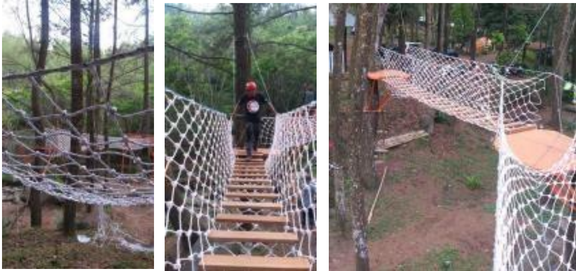
Gambar 7. Pemasangan High Ropes a. Spider Net b. Wood Bridge c. Burma Bridge
